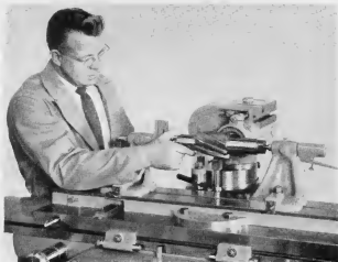
Figure 37A Grinding A Plain Milling Cutter with Helical Teeth
